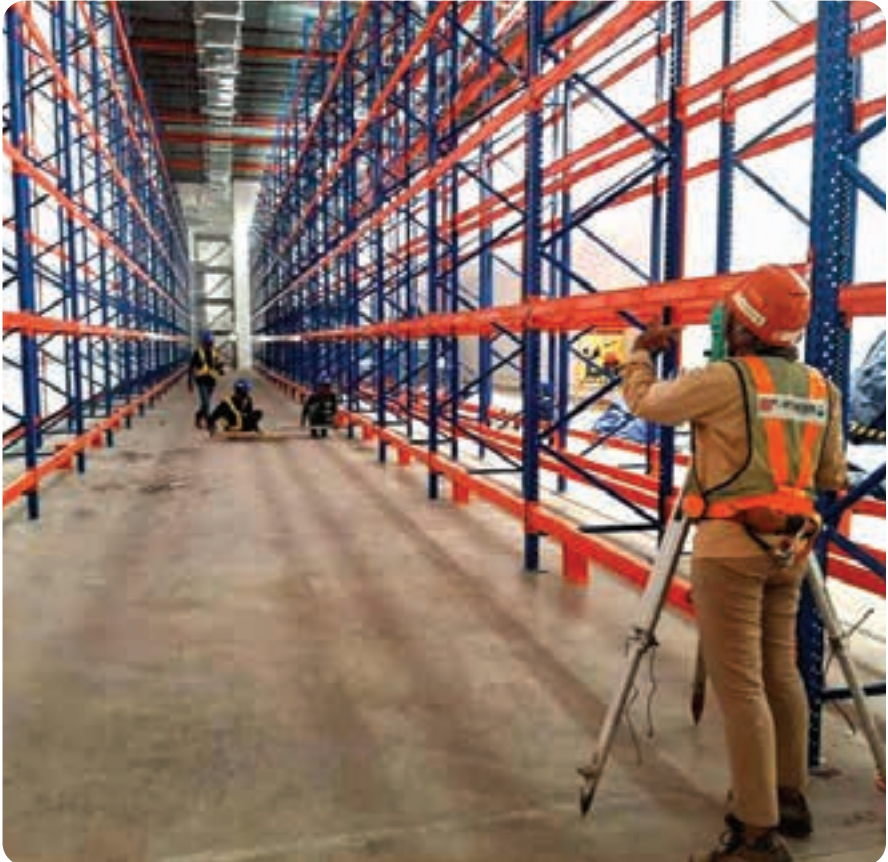
Gambar 1.8 Proses Stake Out
